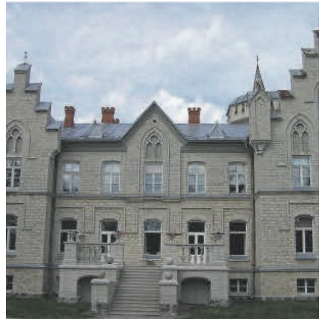
Harju County / Reval limestone facade
