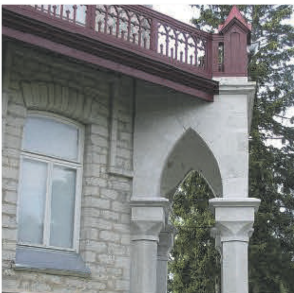
Harju County / Reval limestone facade
